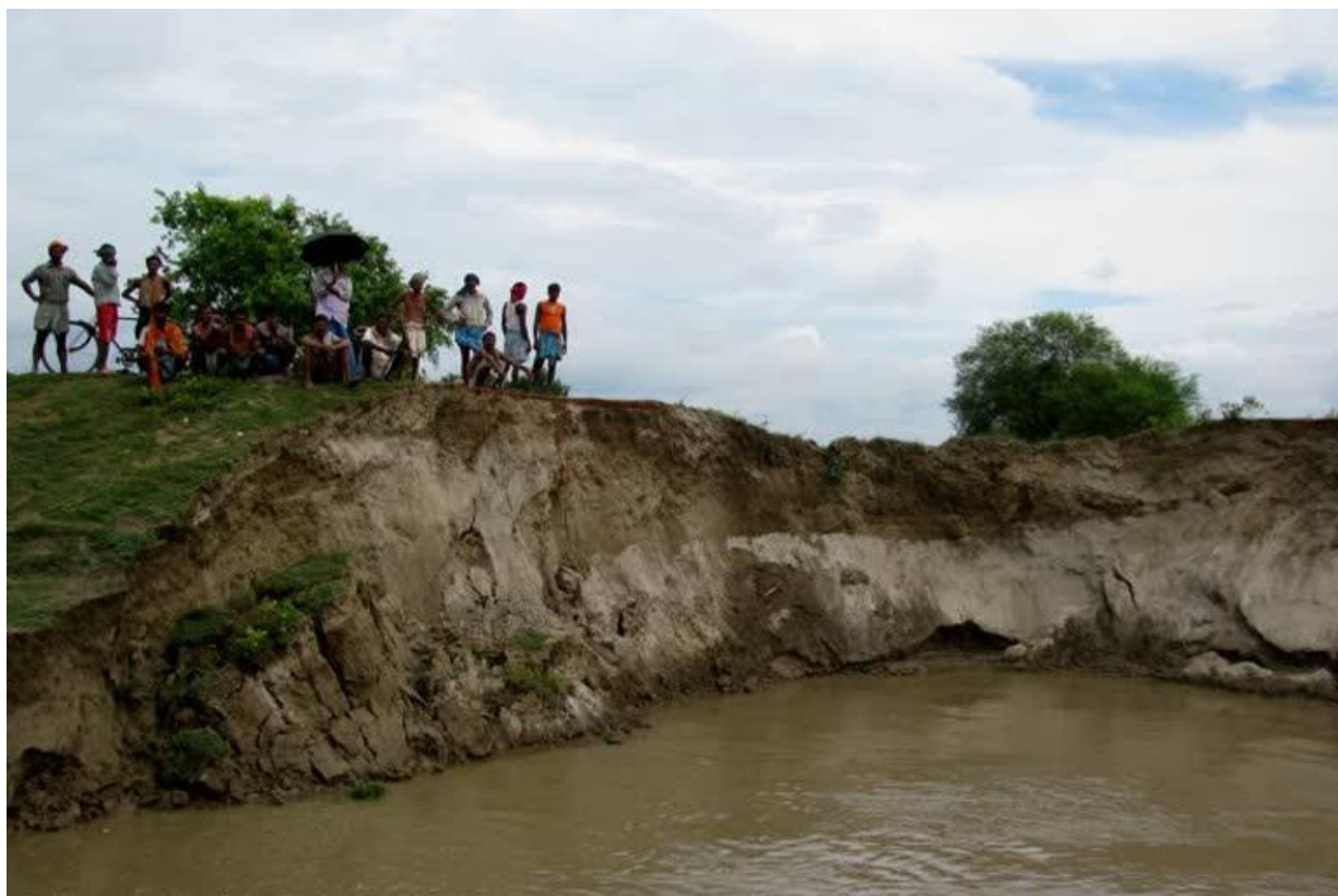
Image No 96 : Bank Erosion at Birnagar G.P, Kaliachak III 24°50'54.10"N 87°57'14.69"E
