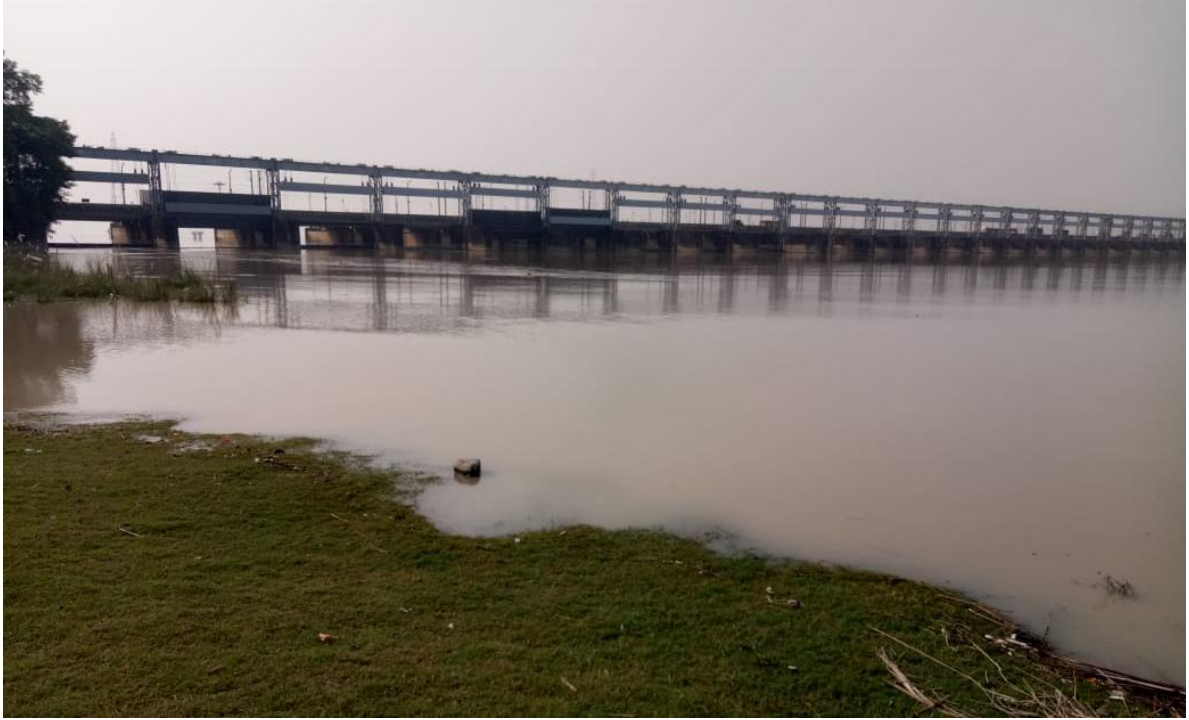
Image No 2 : Farakka Barrage from Lakshmipur, Kaliachak III 24°48'32.47"N 87°56'39.17"E
