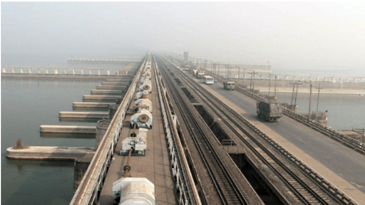
Image No 54 : Farakka Barrage Bridge, 24^{\circ}48'11.68''N 87^{\circ}56'3.55''E
