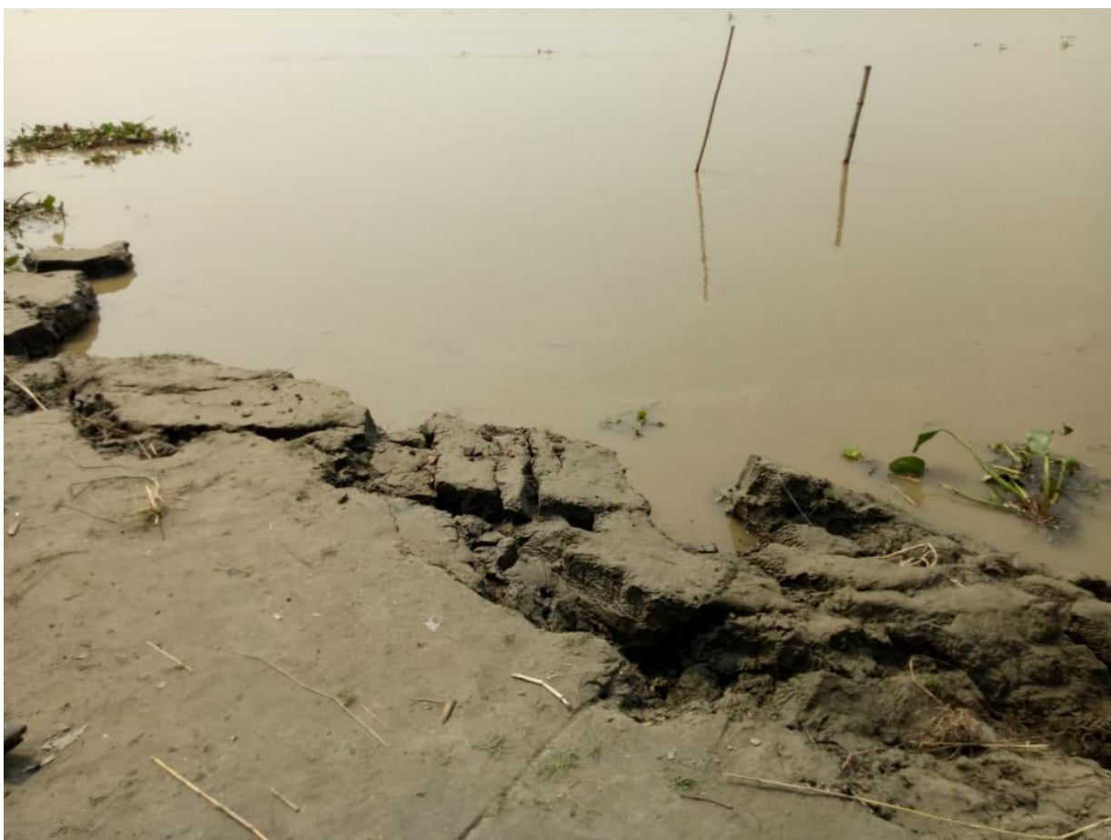
Image No 100 : Collapsing of Banks at Narayanpur Area, Manikchak
