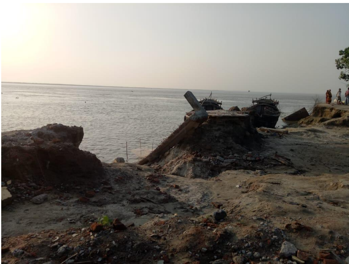
Image No 32 : Extensive Areas are Getting Inundated Because of Channel Shifting, Birnagar G.P, Kaliachak 1, 24°52'44.83"N 87°58'25.36"E
