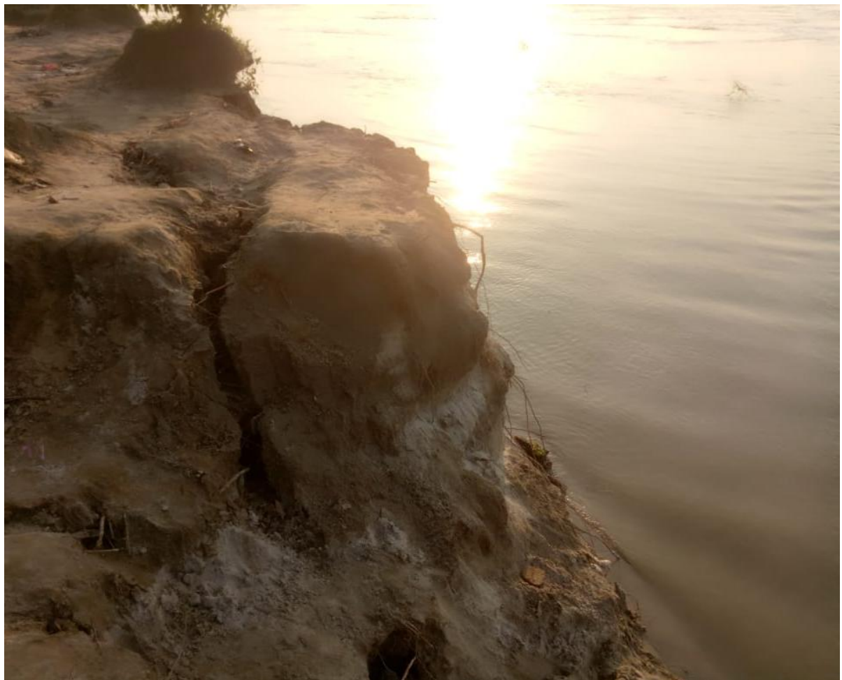
Image No 30 : Active Bank Erosion Area, Panchanandapur
