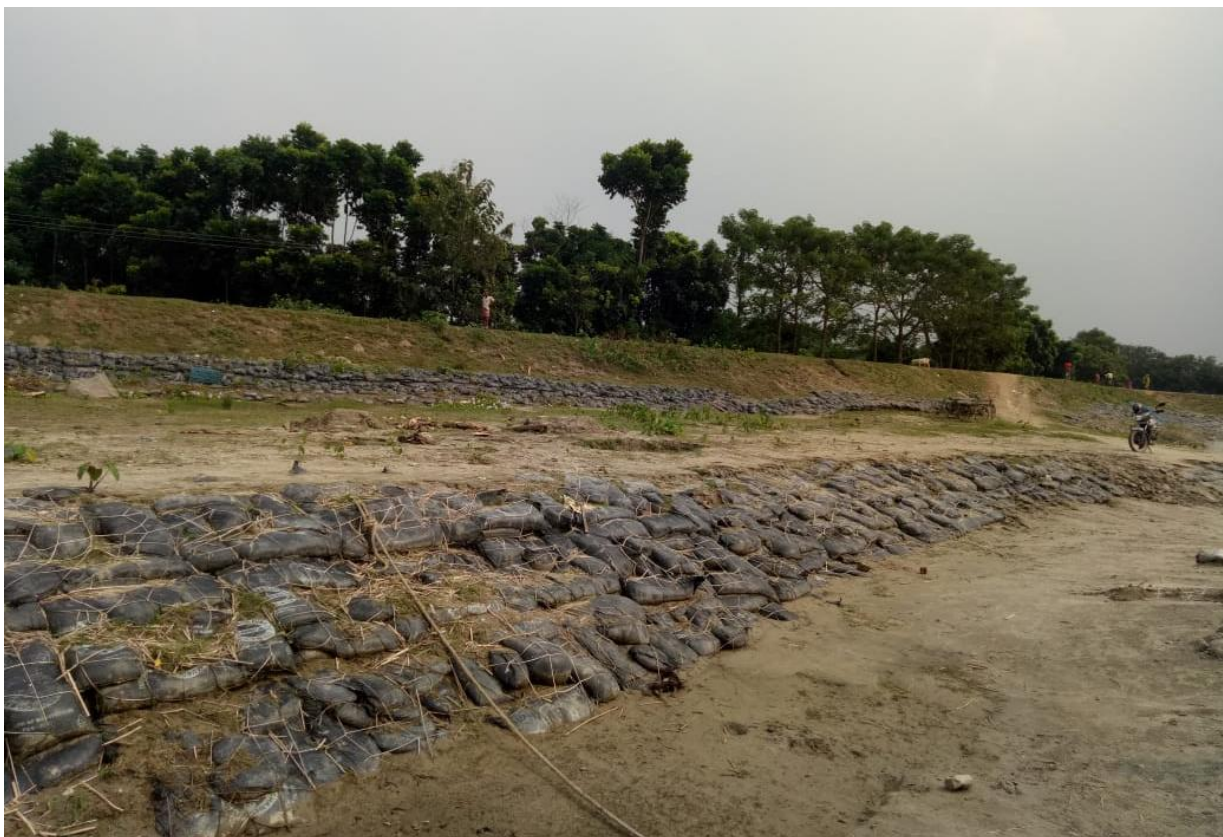
Image No 99 : Sandbags are Used to Protect the Bank Line, Birnagar G.P, Kaliachak
