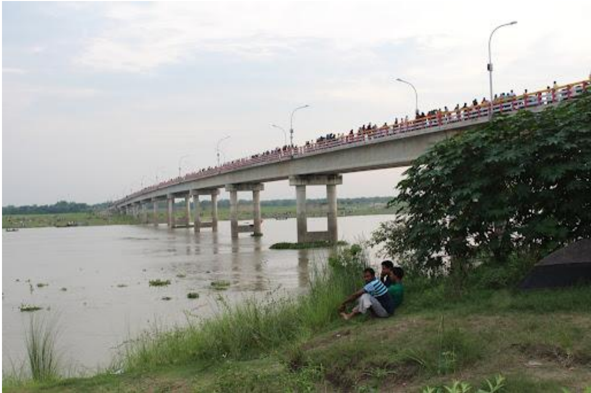
Image No 55 : Mahananda Bridge (2) on Mahanada River 24°59'4.66"N 88° 9'4.07"E
